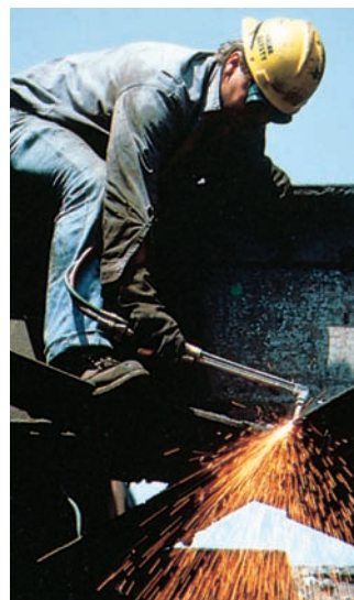
An oxyacetylene torch has a high flame temperature ( 3000^{\circ}\text{C} ) and is used to weld metals.
